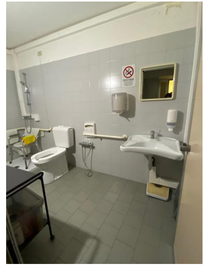
Bagno piano terra
